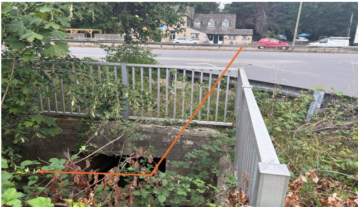
Figure 16 - Rowell Brook A44 culvert outlet with orange flow direction arrow (Site Visit: 2025)
