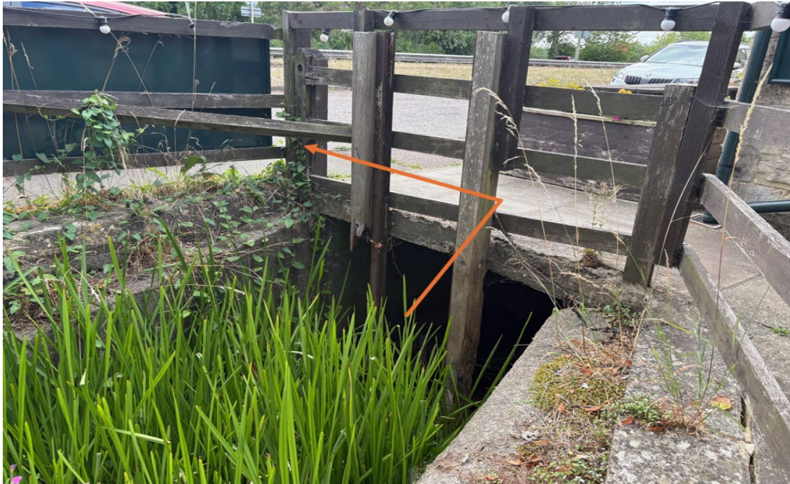
Figure 15 – Rowell Brook A44 culvert inlet with orange flow direction arrow (Site Visit: 2025)
