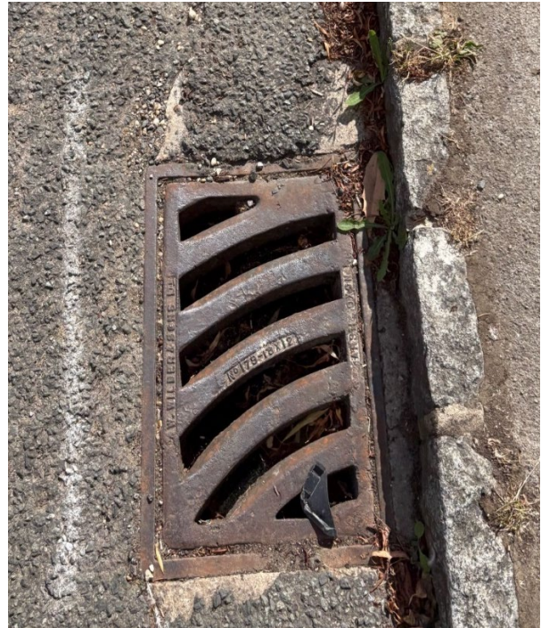
Figure 12 – Drainage infrastructure on Begbroke Lane during site visit (Site Visit: 2025)
